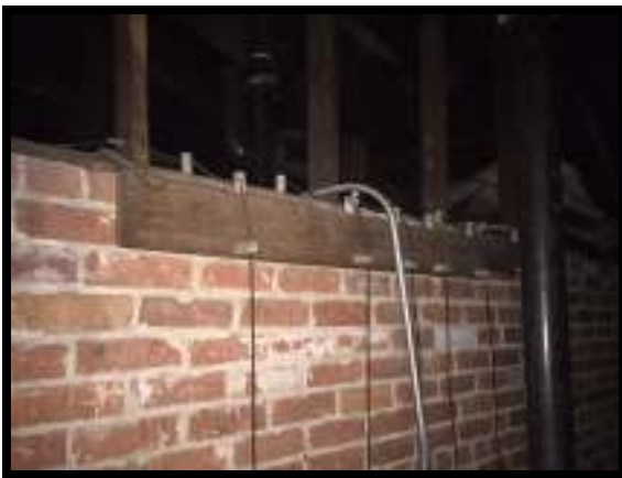
(L) Knob and tube wiring in attic (R) Non-original light fixture in auditorium
