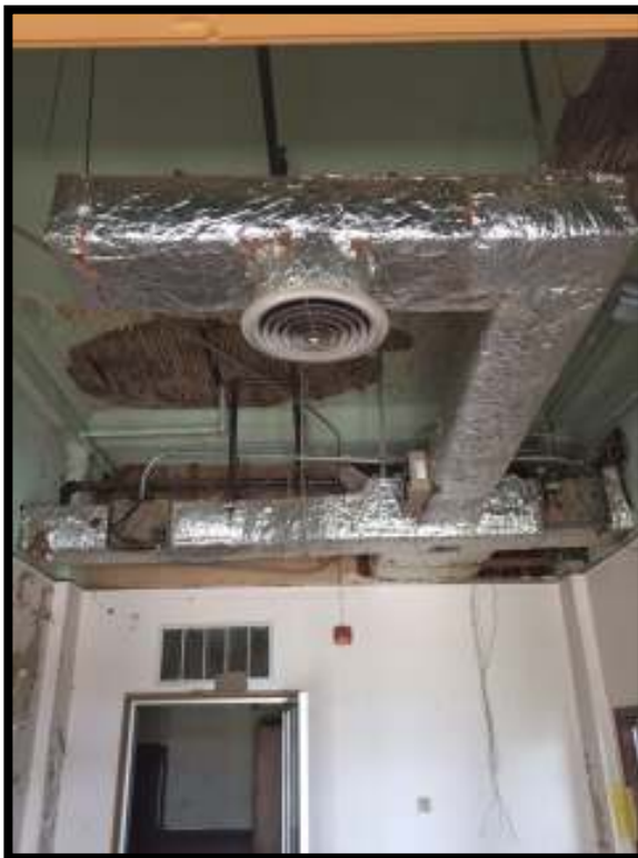
(L) Duct work added to the lobby (R) Ducts in the Auditorium
