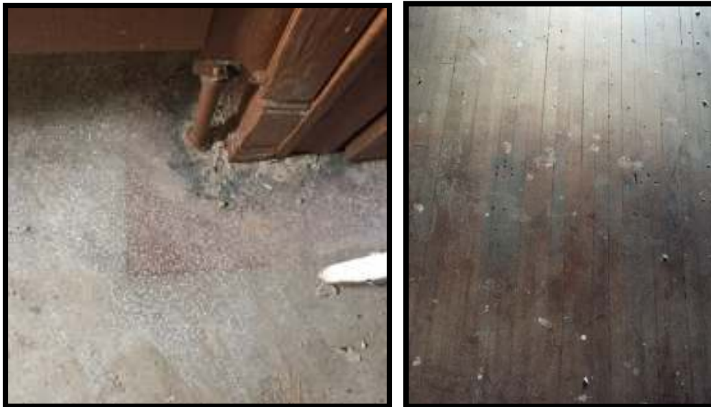
(L) Terrazzo floor with border (R) Wood floor showing mounting and wear pattern of seats
