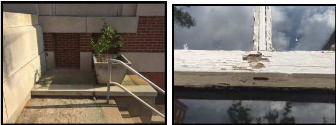
(L) Bricked in basement windows (R) Mortise and tenon construction of original windows
