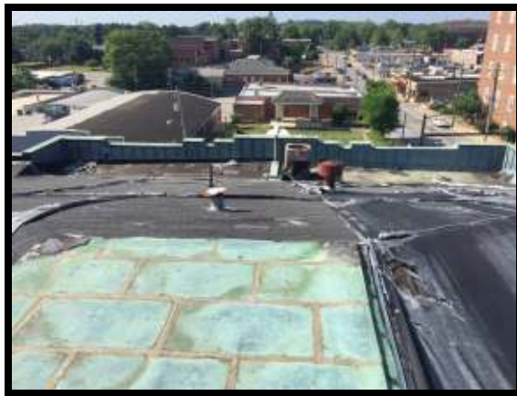
(L) Current roof showing copper plates and ruined tarps (R) Signs or roof leak
