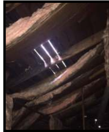
(L) Current roof showing copper plates and ruined tarps (R) Signs or roof leak
