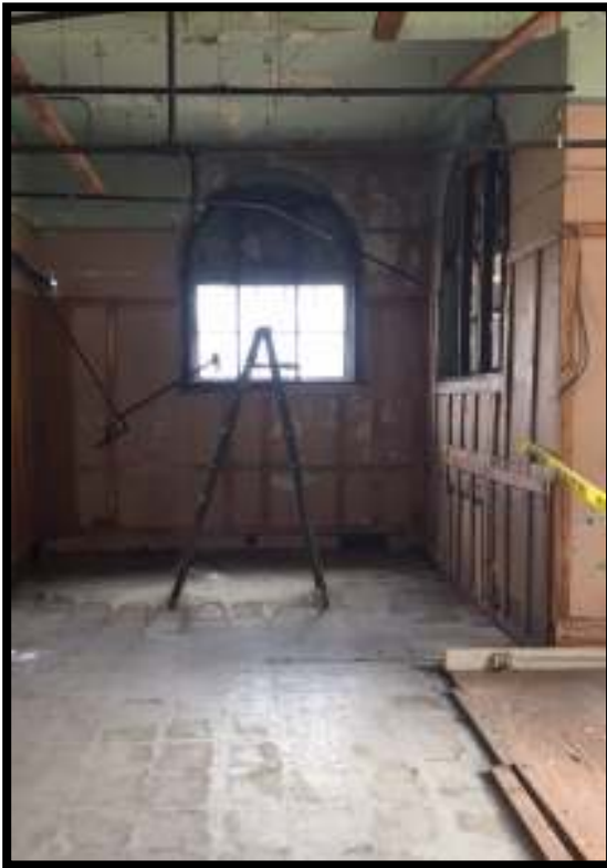
(L) Sprinkler pipes in first floor ceiling (R) Stand pipe in foyer behind door
