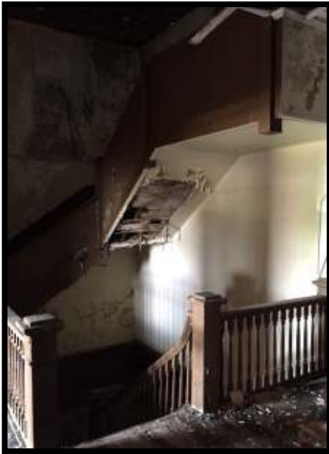
(L) Water damage in surviving stair well (R) Exterior stair well addition in rear
