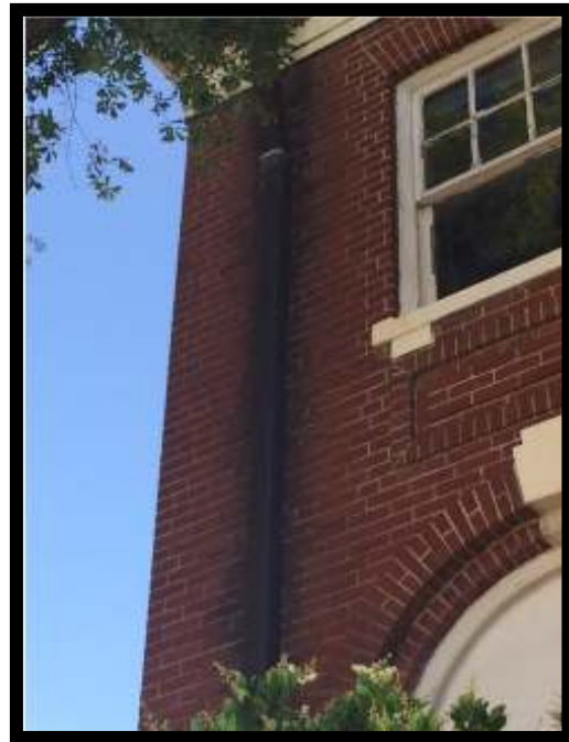
(L) Damage to masonry walls around fire bay doors (R) Signs of overflow eroding brick
